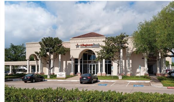
Memorial Spring Branch Office – 8800 Katy Freeway, Houston, TX 77024
